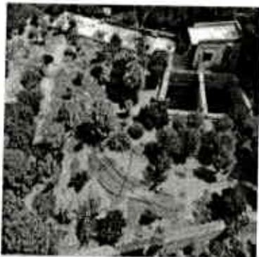
Water Treatment Plant
